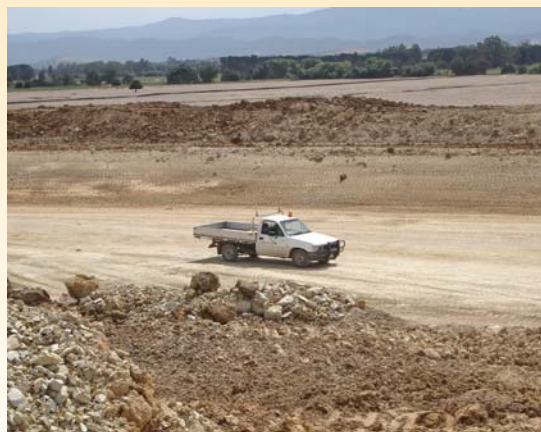
Views of the property looking over the new dam construction.
