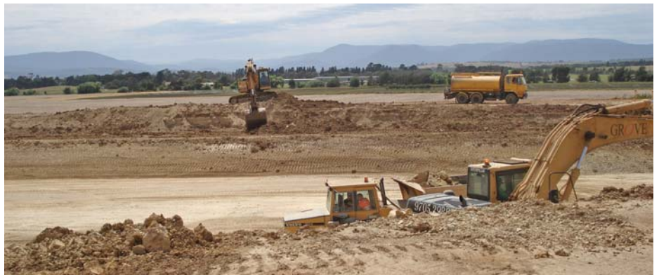
Grove Construction working on the dam.
