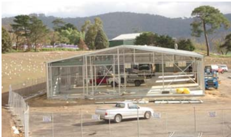
Maintenance Shed under construction
