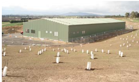
Maintenance Shed June 2007
